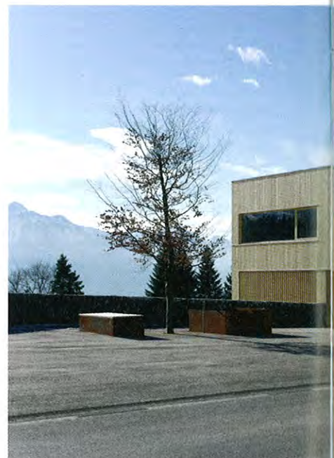
Top right A residential building in Liebefeld, Switzerland by Halle 58 Architects took first prize at the 2010 Passivhaus Architecture Awards (ph: Christine Blaser). Right Joint second prize went to the Saint Gerold Municipal Centre in Austria by Bregenz-based practice Cukrowicz Nachbauer Architects (ph: Hanspeter Schiess).
