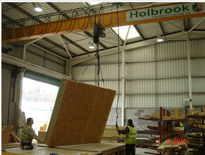
Larch House and Lime House timber frame being assembled © bere:architects
