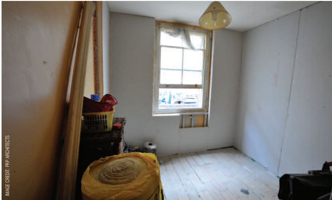
LEFT Aerogel internal wall insulation was specified by PRP Architects at Follett Street in Tower Hamlets, London.
