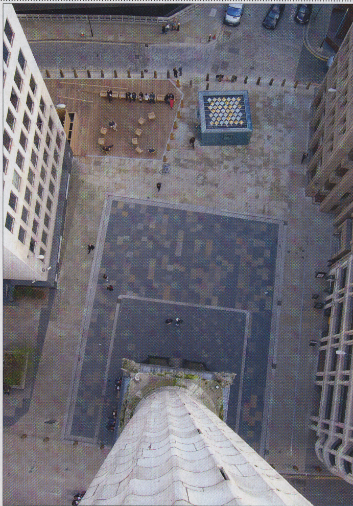
Piazza the action The new-look base, as seen from the top
