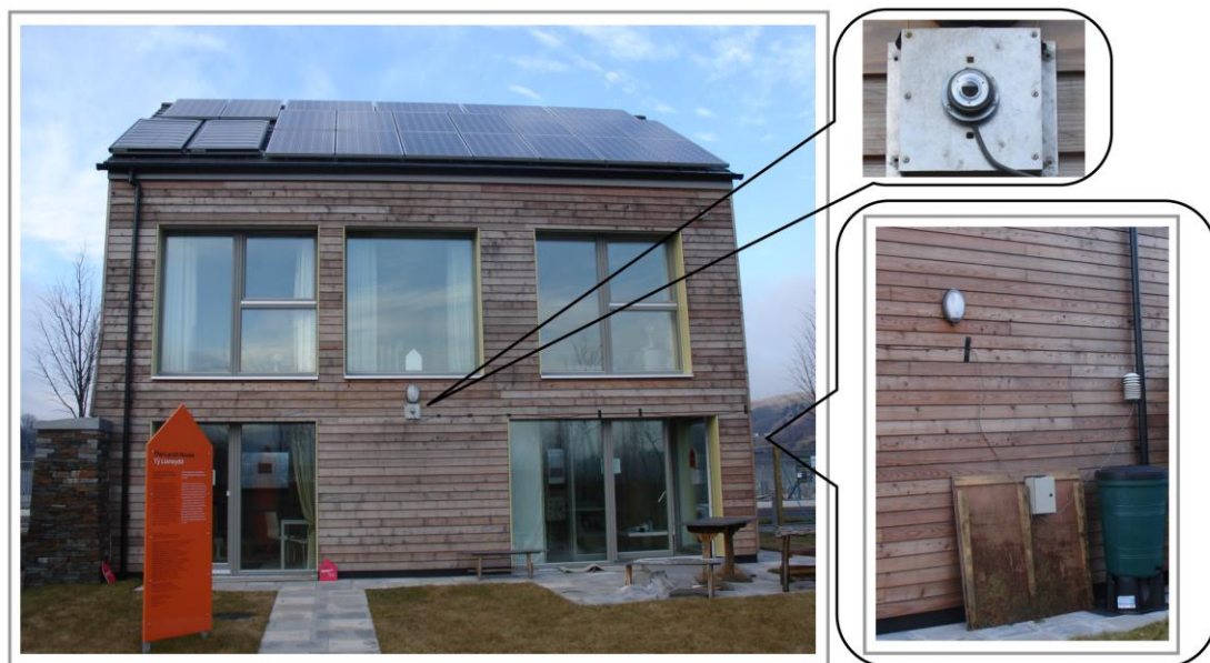
Figure 2.5 Outdoor temperature, relative humidity and solar radiation measurement
