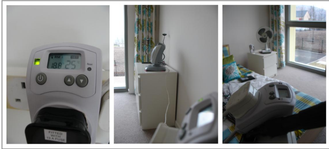
Figure 2.2 Thermostat plug, fan heater and circulation fan
