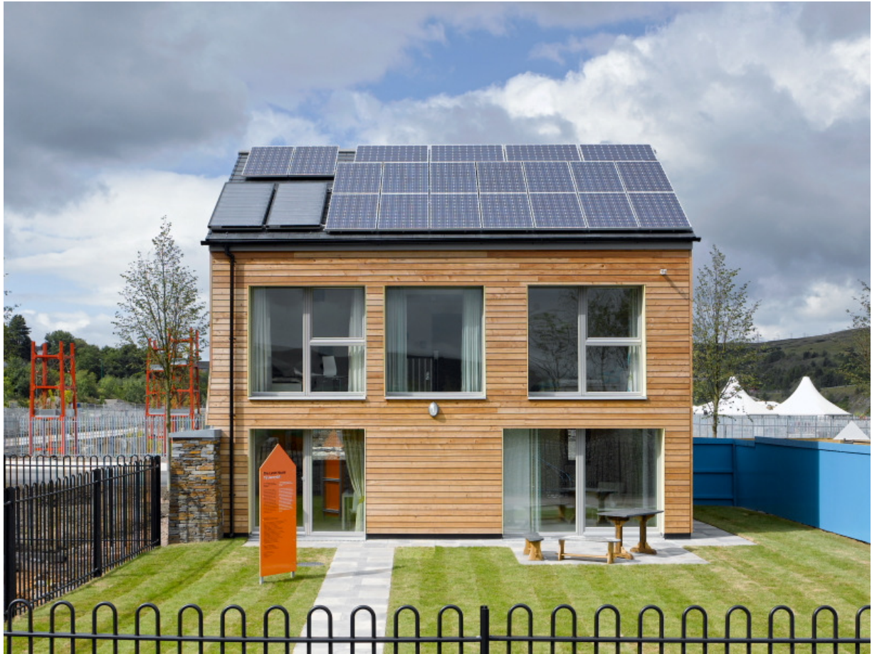
Larch house, Wales' first Code Level 6 house, and its first passive house, when it was still open for visitors
