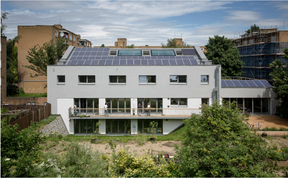
Mayville Community Centre - south elevation - after retrofit
