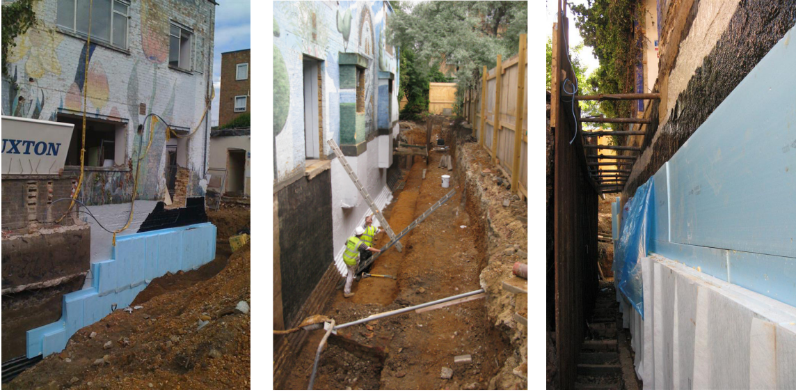
Mayville Community Centre - during construction
